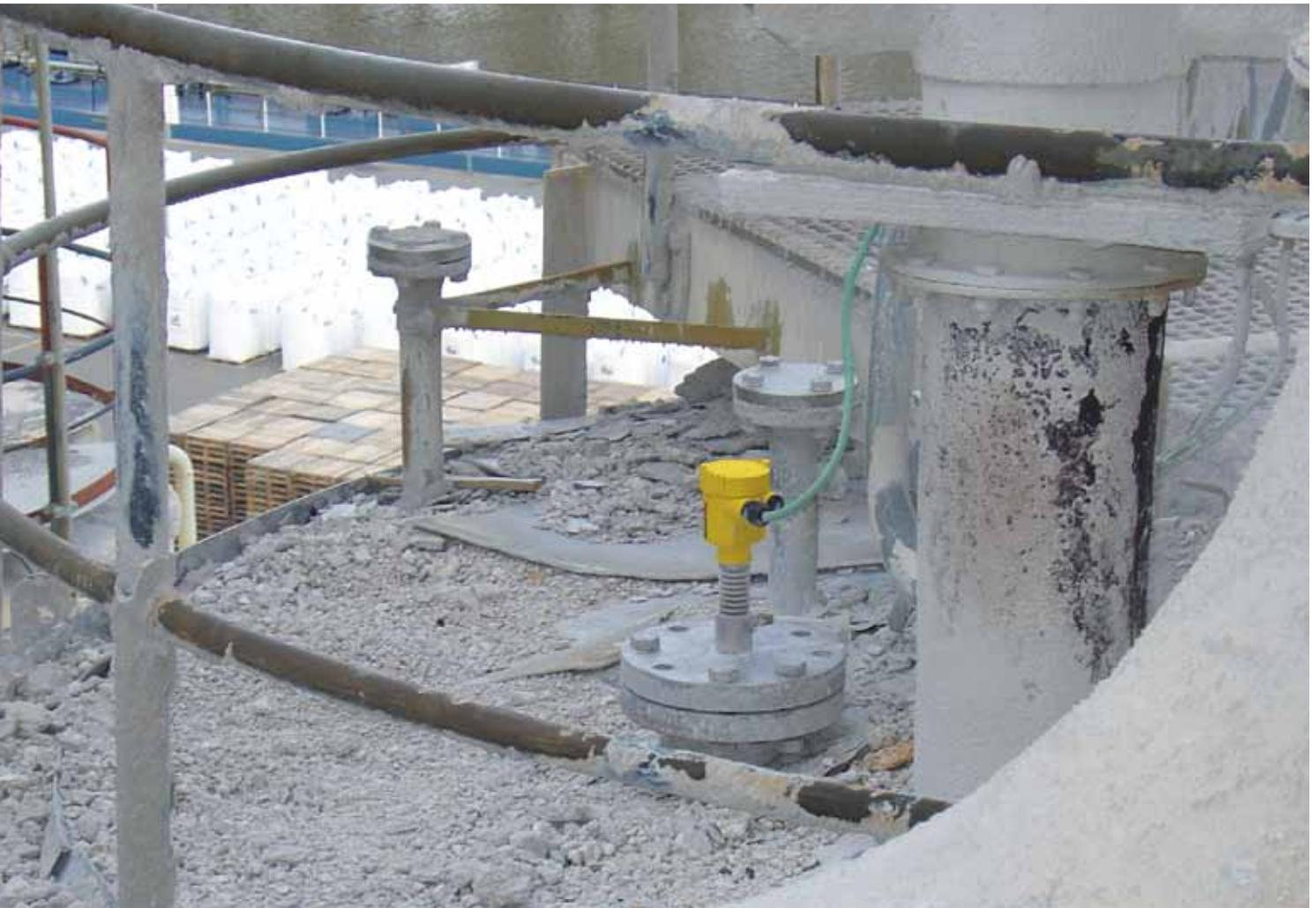
Extreme conditions: Intermediate storage tank with VEGAPULS 68 radar sensor.
