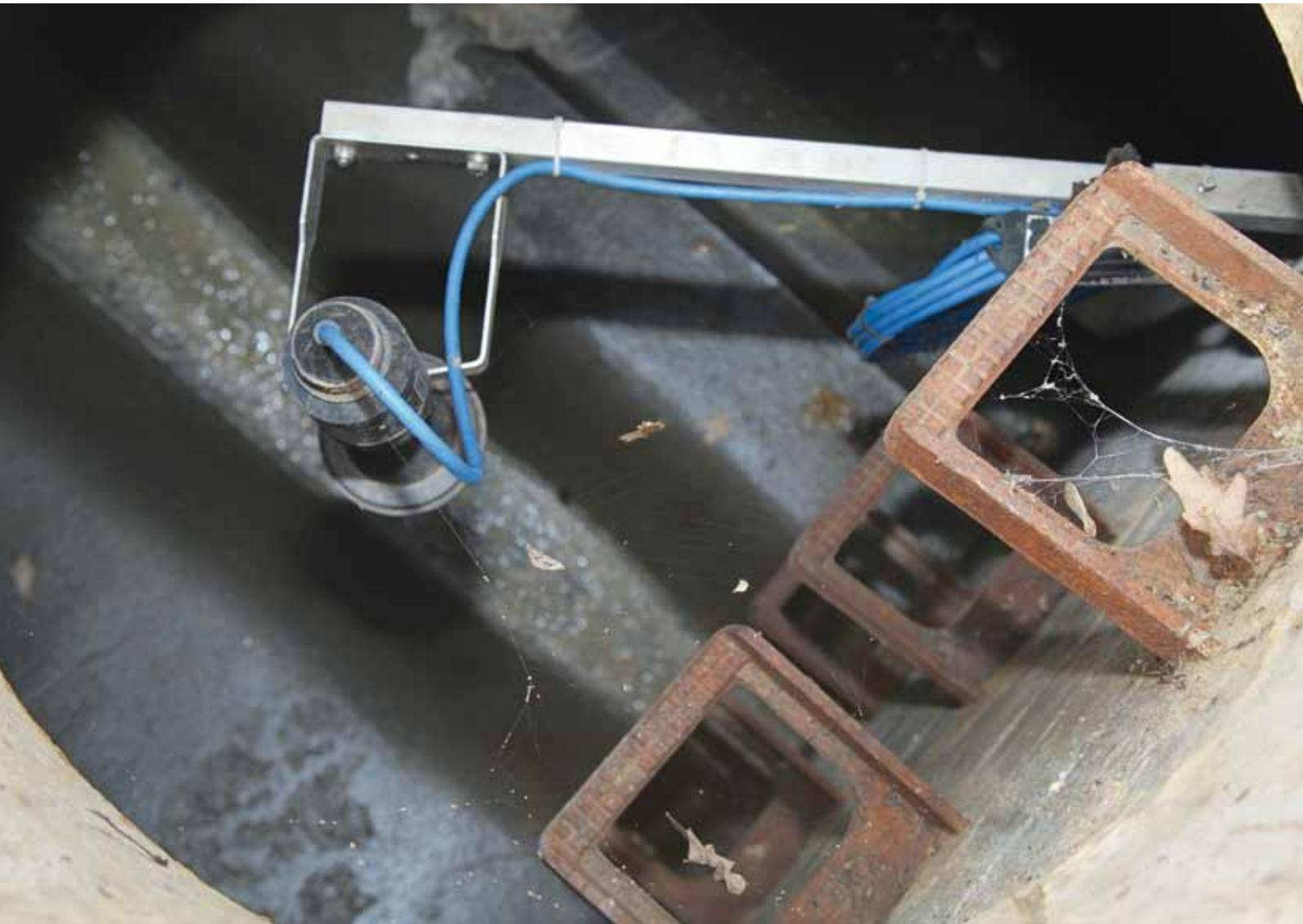
The shaft of the sewage pumping station is located in the middle of a flood-endangered area, so the radar gauges were designed with protection category IP 68.
