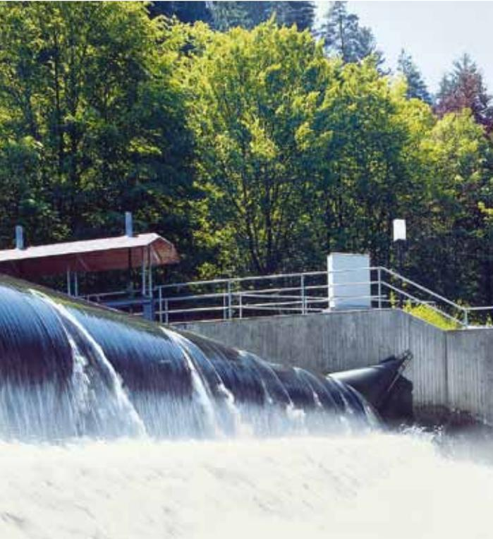
A 250 kW generator in VEGA's hydropower plant in Schiltach has been providing electrical energy for the company since 1997. It generates up to 50 % of the annual electricity requirement.
