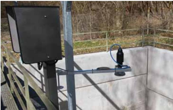
The radar sensor always has its eye on the level in the stormwater basin. A remote control system sends the measurement data to the control room via mobile phone network.
