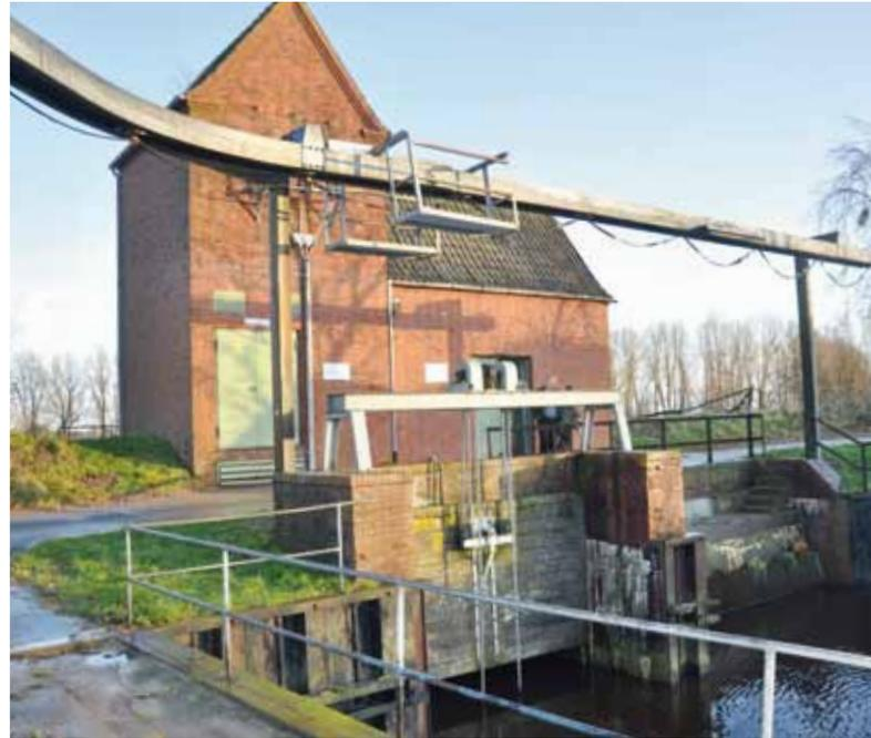
The pumping station at Tielenu is used to drain the middle reaches of the river Eider. The total capacity of the pumps is 6 m<sup>3</sup>/s.
